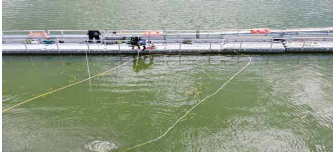
Council workers reattaching the Malpas Dam pontoon to its moorings. The pontoon broke loose last year.
