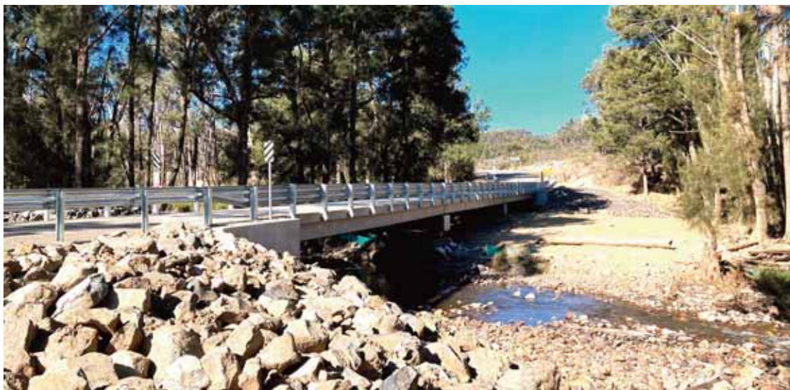
The recently completed Laura Creek Bridge
